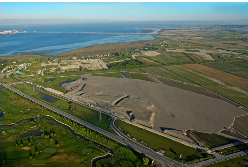
Ariel Photo of the Commercial Lands fill site
