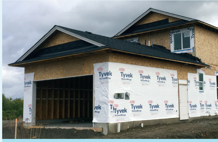
A Member's home under construction on Falcon Way.
