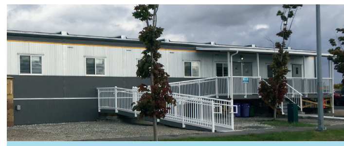
The Lands Department's temporary office space on Falcon Way.
