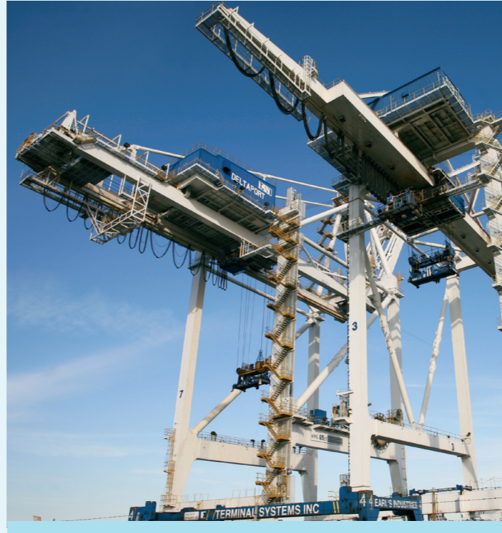
Ship-to-shore container cranes at Roberts Bank.
