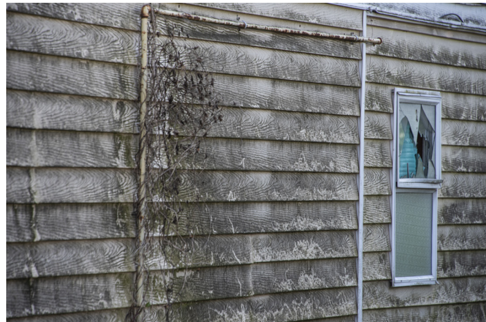
This previously white home on TFN Lands is covered in diesel particulates, which has affected several homes on TFN Lands. Many photos like this were presented to the Review Panel.
