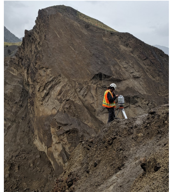
LIDAR technology is instrumental to site safety.
