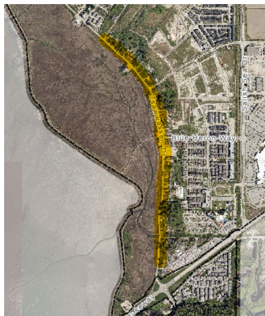
Figure 1 – Stretch of Tsawwassen Drive requiring roving single-lane alternating traffic for drainage maintenance of select driveway entrances
